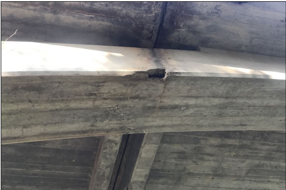
Span 2 right arch rib has spall with exposed rebar near mid span.
