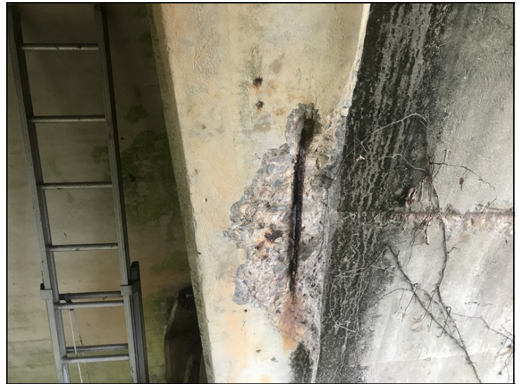
Bent 1 left column exposed reinforcing steel with section loss.
