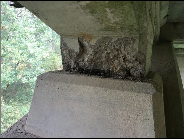
Span 2 spandrel column 2 on rib 1, spall with exposed reinforcing steel.
