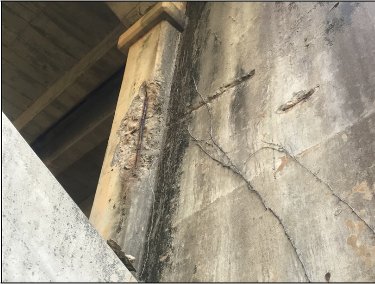
Bent 1 left arch spandrel column 1 has spall with exposed rebar.
