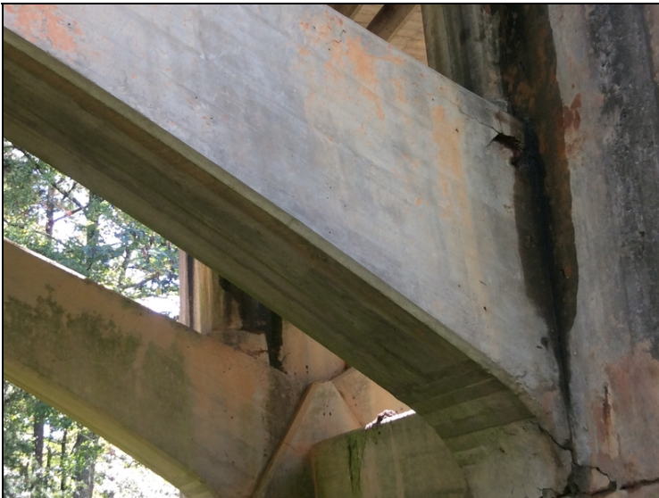
Span 2 left arch spall with exposed rebar
