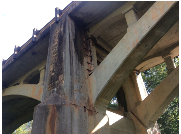
Bent 2 exposed rebar.
