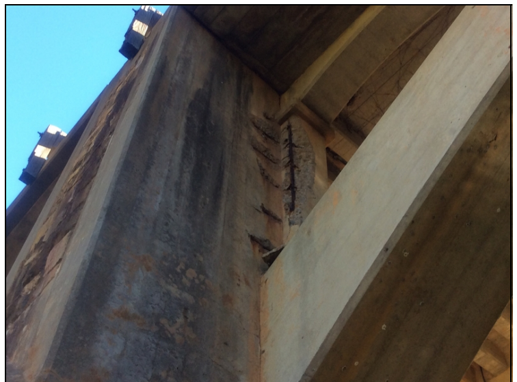
Exposed rebar
