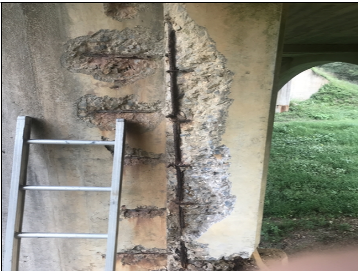
Bent 2 spandrel column left side, spall with exposed reinforcing steel with section loss.
