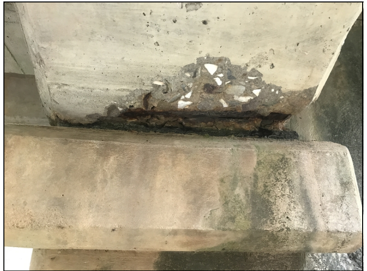
Bent 2 right side spall at bearing area with exposed reinforcing steel.
