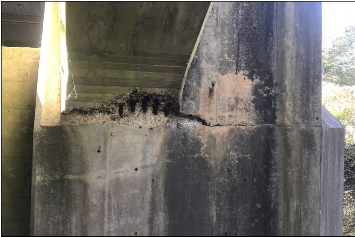
Span 2 bottom of left arch rib has spall with exposed rebar.
