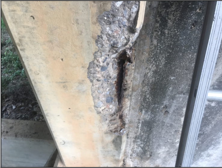
Bent 2 right spandrel column spall with exposed reinforcing steel and section loss.
