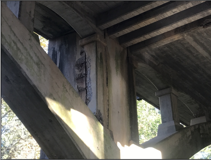
Span 1 Spandrel column left side at bent 2 has spalls with exposed rebar.
