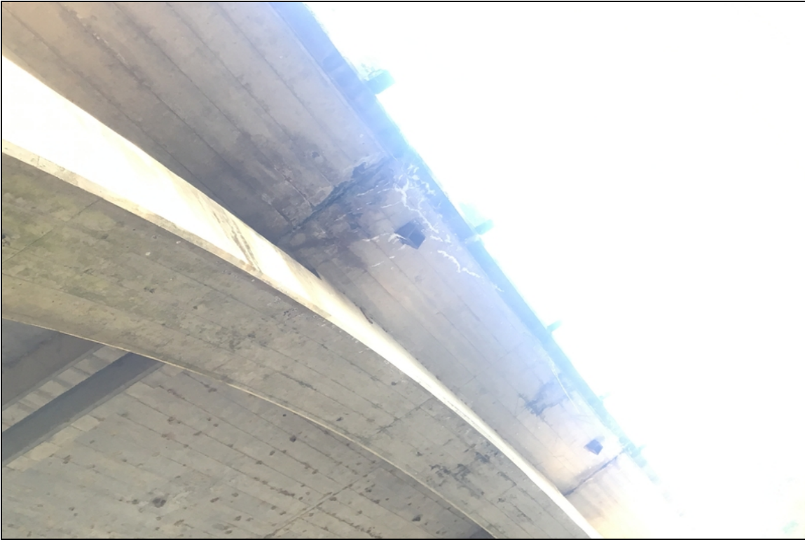
Span 1 right side soffit overhang has cracks with efflorescence.
