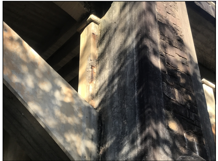
Span 1 right side at bent 2 spandrel column has spall with exposed rebar.
